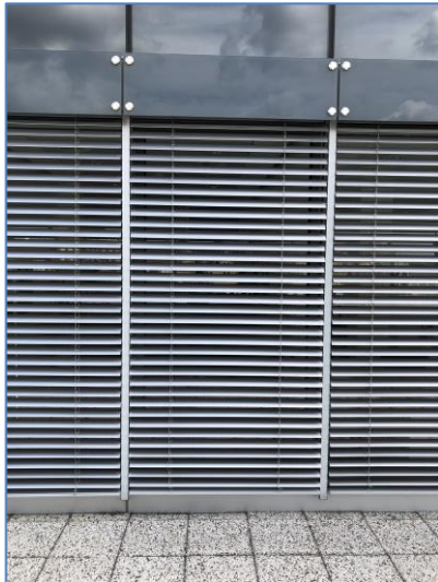
Figure 25: External sun protection
