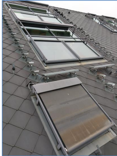
Figure 26: External sun protection barracks
