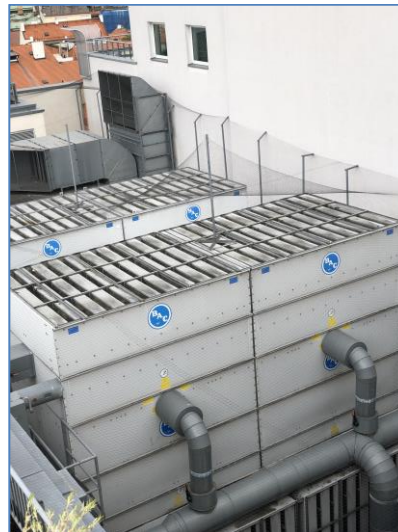
Figure 24: Cooling Tower
